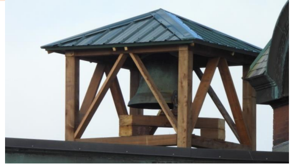
The Bell Tower following reconstruction November 2023. Photo courtesy of Tammey McLean.
